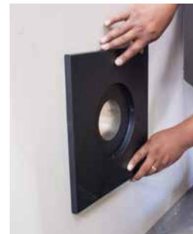
6. Level and attach inside portion of the wall thimble to the wall.
