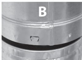
Assemble the gas vent sections.
