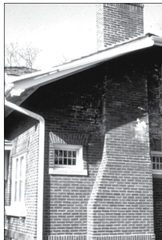
Spalling bricks
