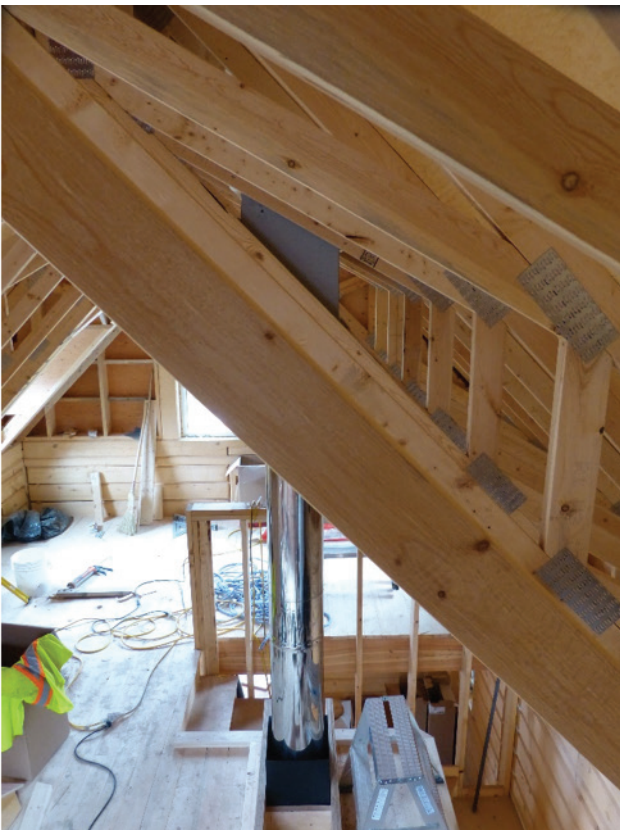
Pass-Through Radiation Shield in place within truss assembly
